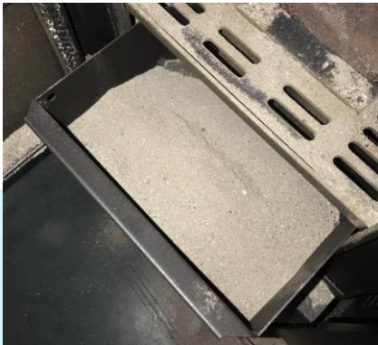
Example of dirty ash box
